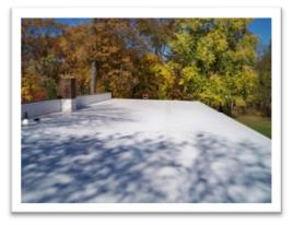
The temperature of your roof affects the temperature inside your building. White roofs, cooling shingles, and other materials with advanced reflectivity can be 40 percent cooler than traditional dark colored roofing material. The sun's heat is reflected back instead of being absorbed into the building, resulting in energy savings by decreasing cooling costs.
